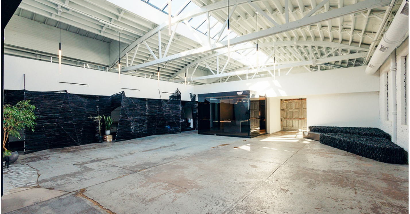
INTERIOR Clear-span bow-truss structure with 75' operable skylight
